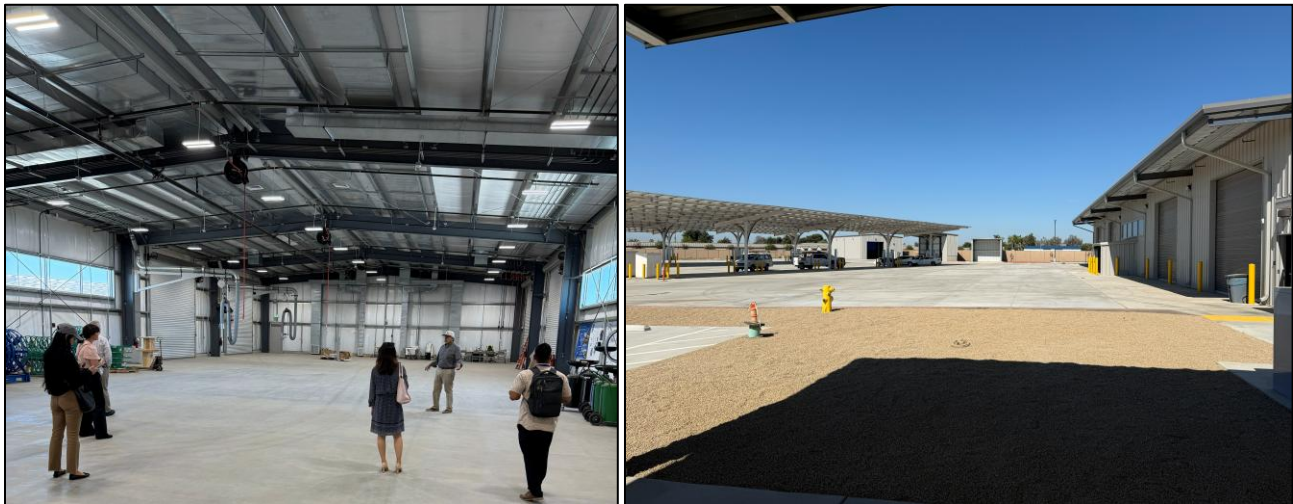
Figure 6 FCRTA's Selma Maintenance Facility
